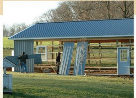
Installing Metal Siding
