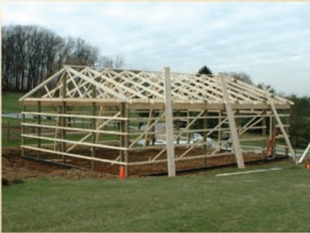
Framing and Setting Trusses
