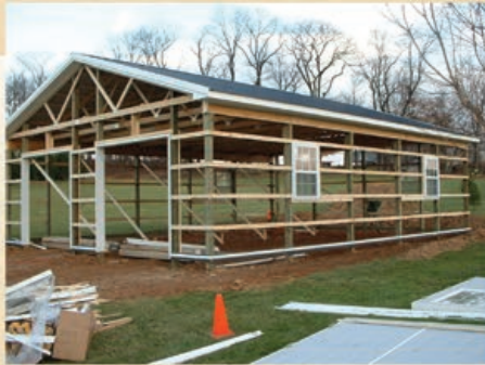
Installing Metal Roof
