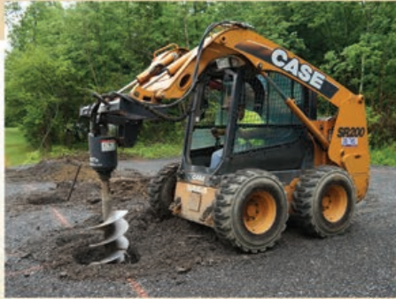
Drilling Post Holes
